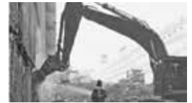
DEMOLITION / CONCRETE / BUILDING RENOVATION
